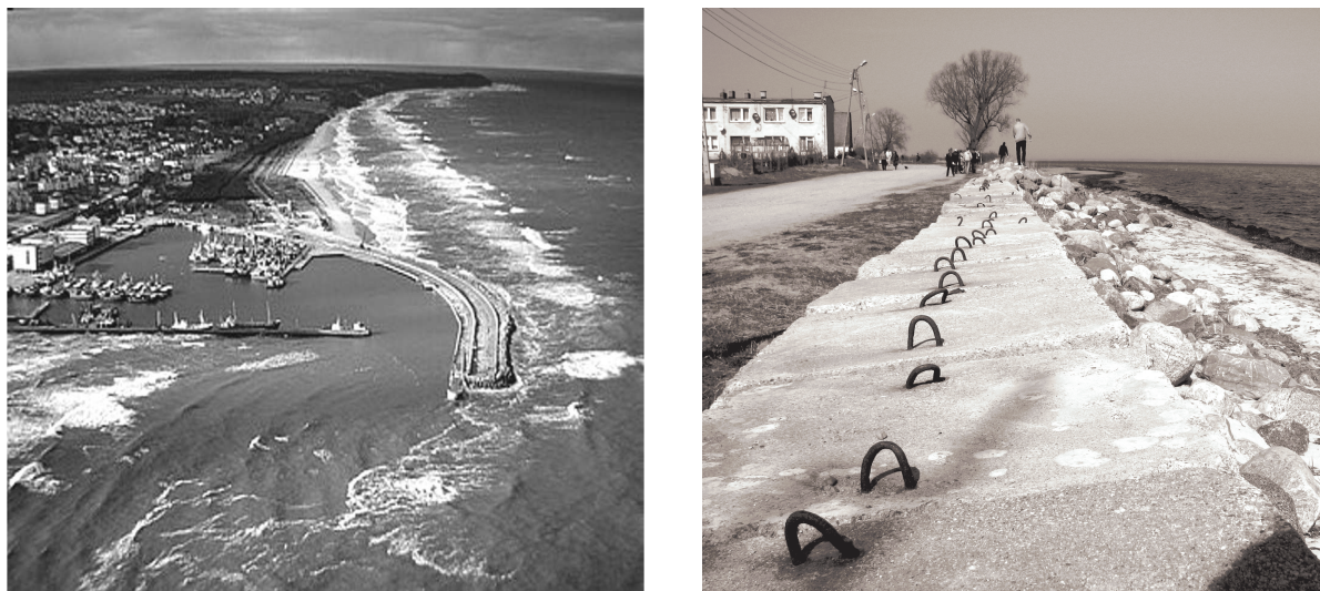
Fig. 8. Examples of coastal “hard” constructions: Władysławowo fishing port (left) (www photo) and concrete wall in the Puck Bay (right).
